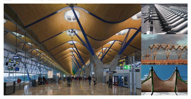
The 125,000 m2 occupied by the Terminal Building of the new terminal of Barajas Airport are distributed between a central zone of  $360,00 \times 216,00 \text{ m}$  on plan and two lateral dike-like constructions of  $396,00 \times 54,00 \text{ m}$ . Depending on the area, these dike-like constructions have up to three underground levels and two over ground ones.
